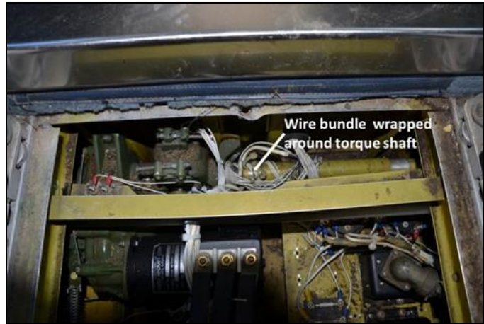
Photo 2. Wire bundle wrapped around the landing-gear torque shaft
