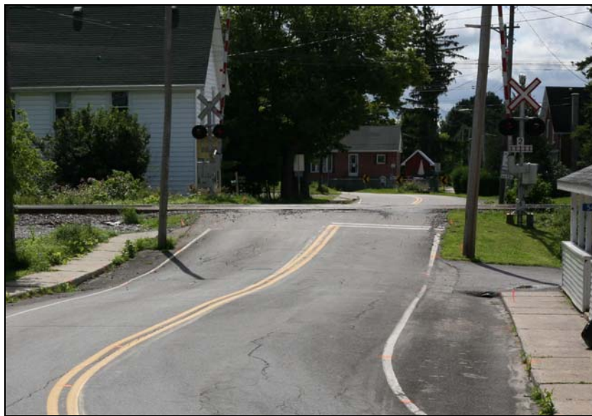
Photo 2. View of the Quabbin Road crossing looking south
