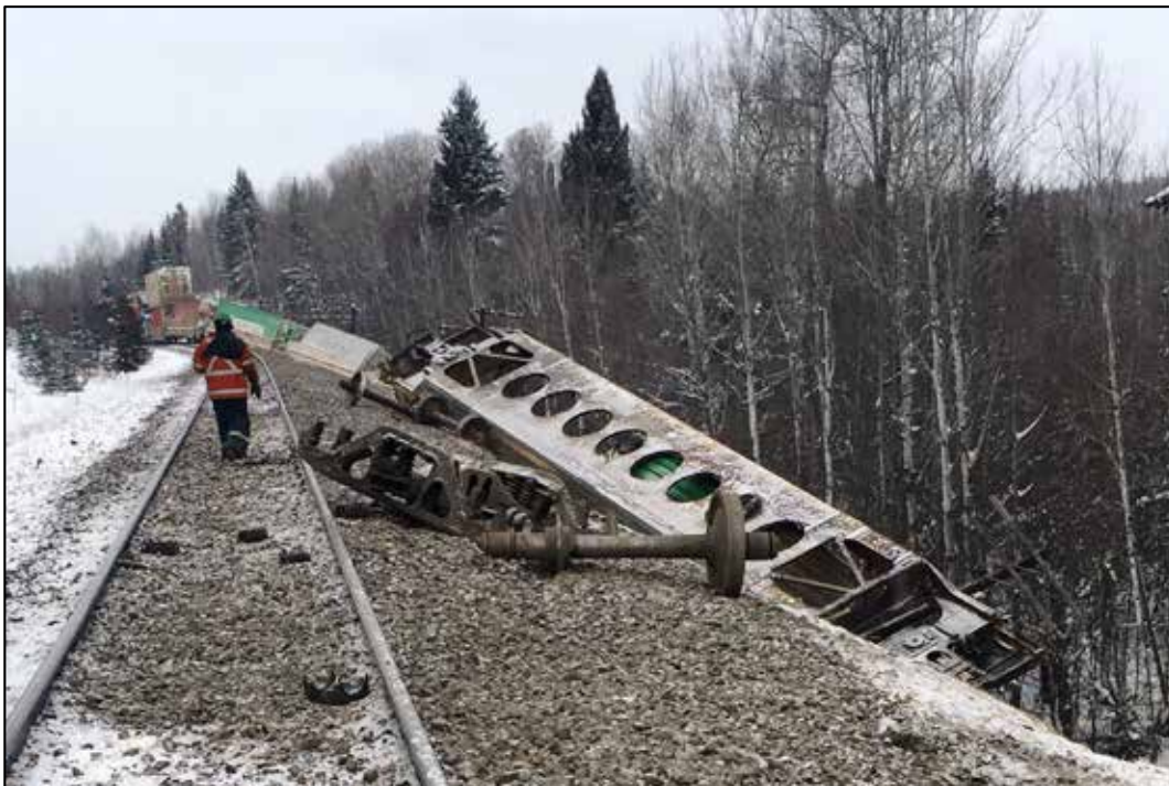
Photo 1. First 2 derailed cars and broken wheel set (Source: Canadian National Railway Company)
