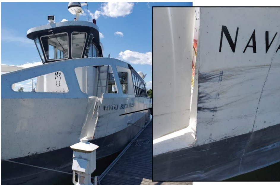
Figure 7. Damage near the Navark Faucon Millenium 's forward access gate (Source: TSB)
