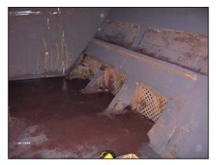
Photo 5. Strainer plates in the aft port cargo hold
