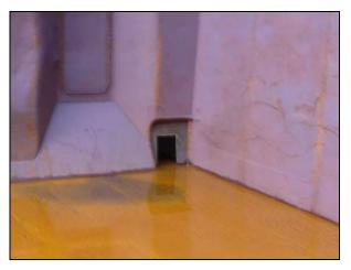
Photo 4. Screen bulkhead drainage opening
