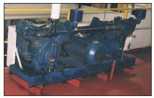
Photo 14. Air compressor arrangement showing electrical motor between two compressors
