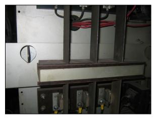
**Photo 7.** Side view of a standard arrangement of the three vertical bus bars resting in bakelite insulation and encased by the steel bracket
