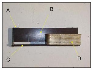
Photo 8. A. Steel bracket. B. Horizontal bakelite insulation block with the three notches.C. Vertical 6 mm flat bakelite insulation piece. D. Bus bar in the centre notch.
