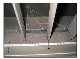
Photo 10. View from above of: A. Three bus bars.B. The bakelite insulation block.C. Indication of arcing in way of the bus bars.
