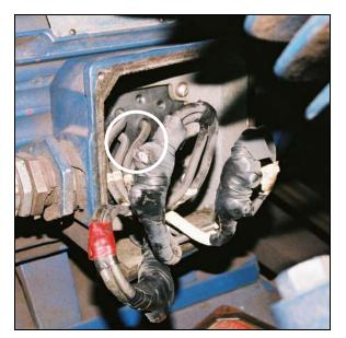
**Photo 15.** Wire terminal covered with electrical tape, but showing bare screw
