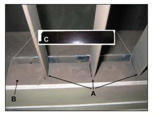
Photo 11. View from above of: A. Three bus bars.B. The bakelite insulation block.C. Normal location of the 6 mm flat bakelite insulation piece (insert).
