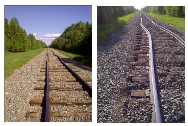
Photo 1. Eastward view showing the track buckle (north is to the left)
