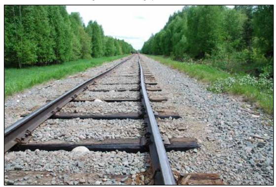
Photo 5. Ballast and rail anchoring conditions leading up to the derailment site
