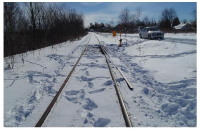
Figure 1. Split switch derail at Mile 46.19 looking eastward (Source: TSB)
